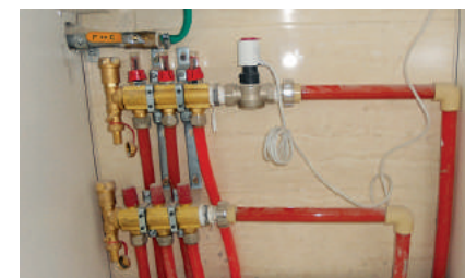
Danfoss manifold with RA-G valve and TWA-A actuator. This combination was installed in the smaller apartments to provide central temperature control via a CWD thermostat in the main living room. Individual room controls were installed in the larger apartments.
