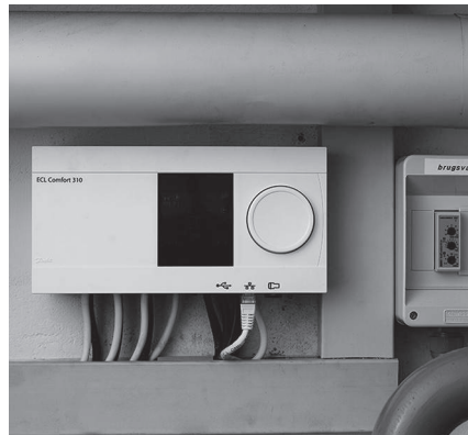
District Heating Controls
